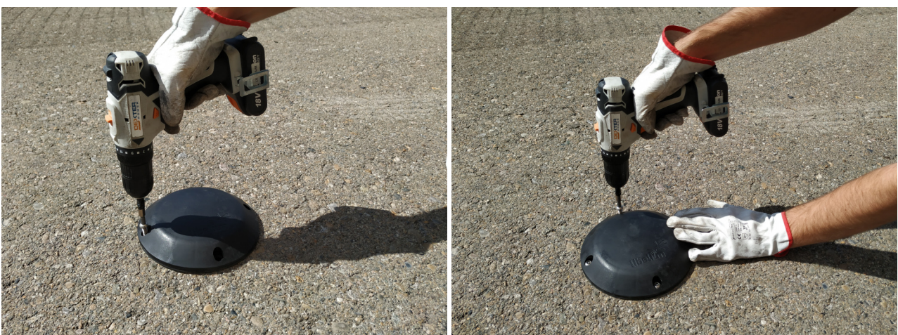
Figure : Screw the node
