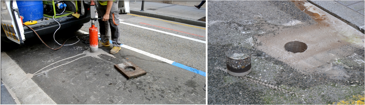
Figure : Making a hole in the pavement
