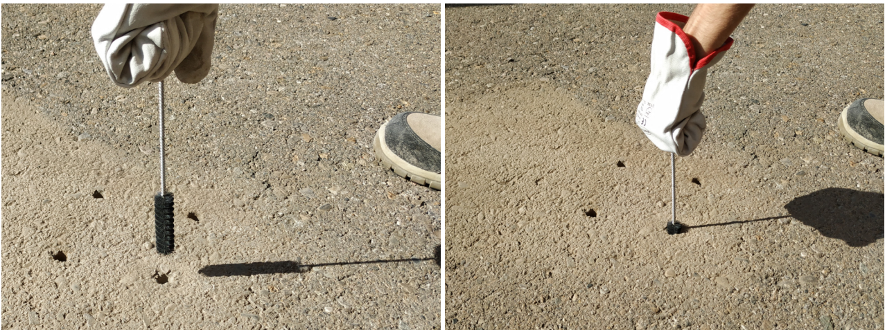
Figure : Brush the hole (step 3)
