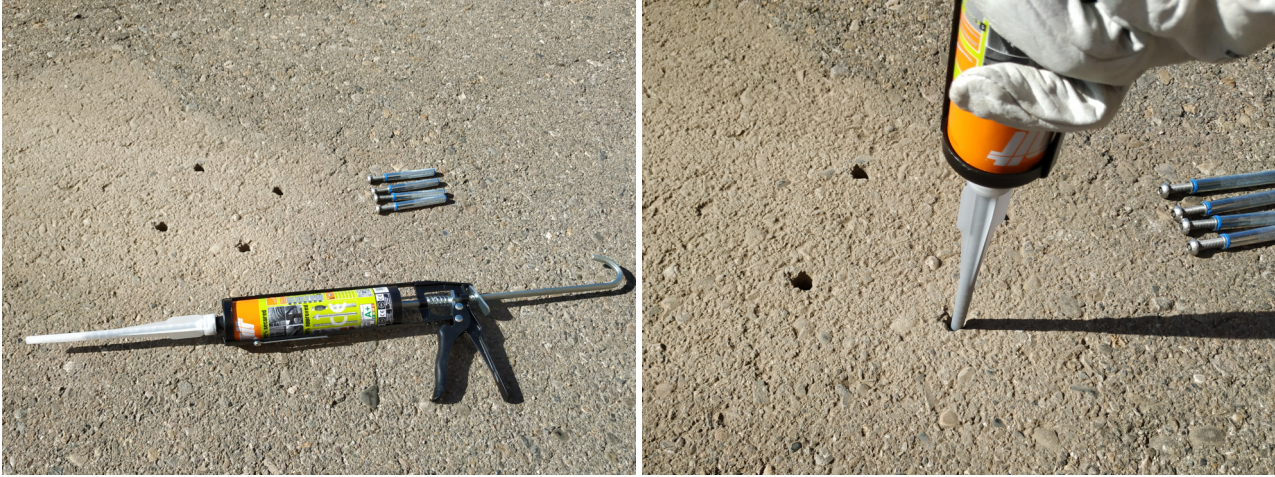
Figure : Inject chemical fixing adhesive (step 5)
