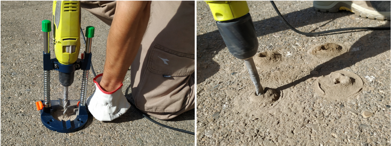
Figure : Drill the holes (step 1)
