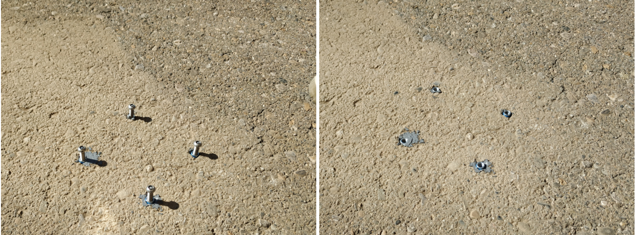
Figure : Final anchor installation (step 7)
