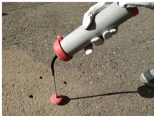
Figure : Blow out dust and loose materials (steps 2 and 4)
