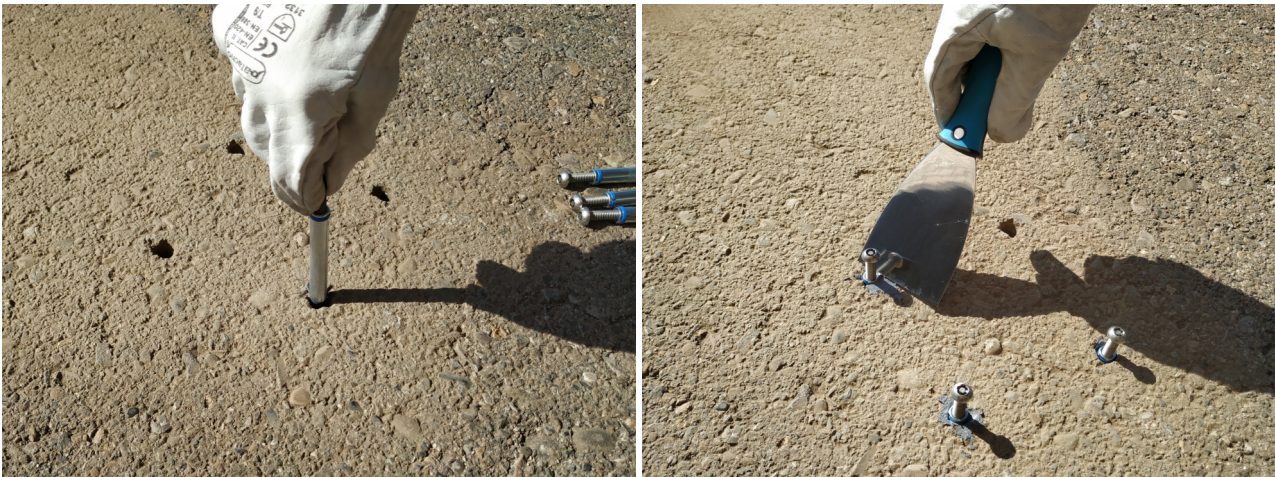
Figure : Insert the anchors (step 6)
